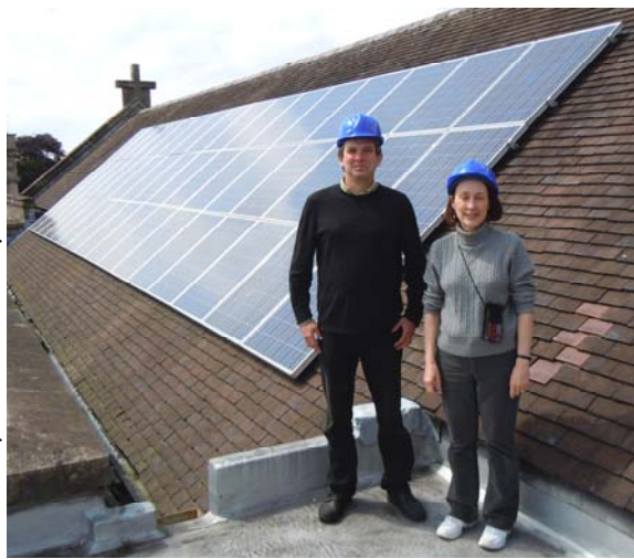
Rev. Stephen Lewis and Rev. Marty Black don their hard hats and inspect the solar panels on top of Redland Park United Reformed Church in Bristol, England.
